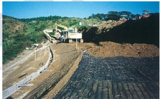
Fig3: Geogrid for Embankment
