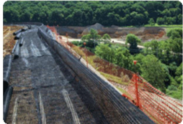
**Fig 5: Geogrid for Slope Protection**
