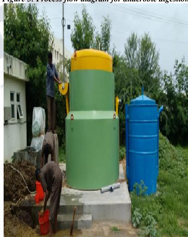
Figure 6: Bapuji Institute of Engineering & Technology installing 6m<sup>3</sup> with 2 tones capacity biogas plant in progress
